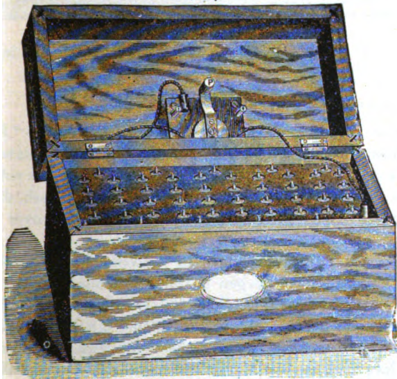
CHLORIDE OF SILVER BATTERY.
