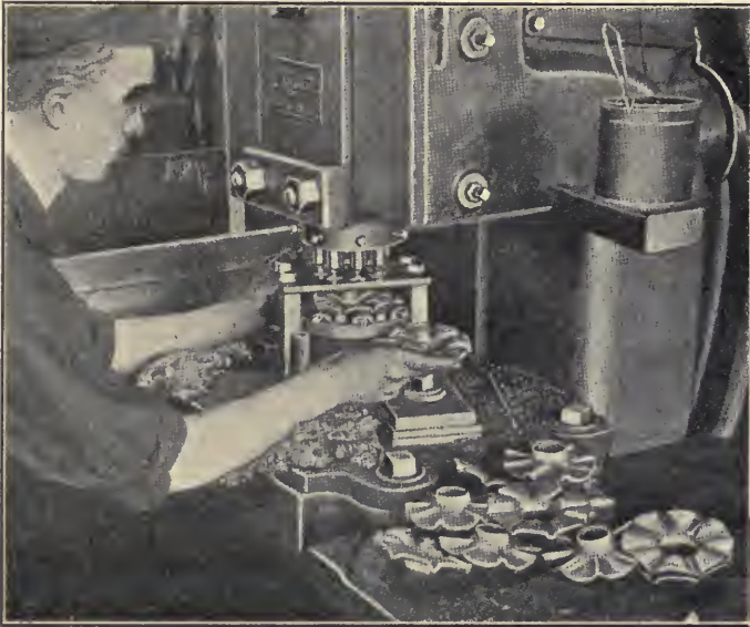
FIG. 208.—Punching eight rivet-holes in flanges.
