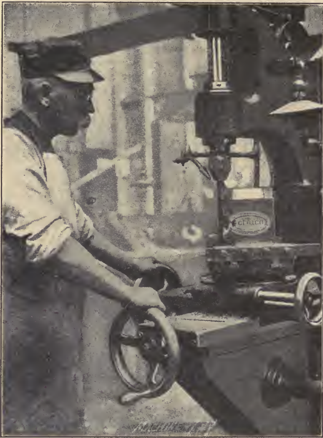
FIG. 4.—Finishing die, Fig. 2, on the profiling machine, Fig. 3.
