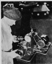
Grinding Cutters on 375-1 Cutter Grinder
