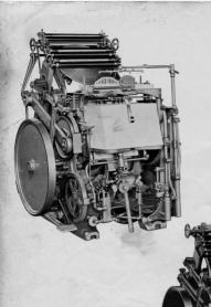
The Chandler & Price Craftsman Automatic Unit 12 x 18 shown here with Micromatic Ink Distributor placed on Units Numbered RD 1649 and up
