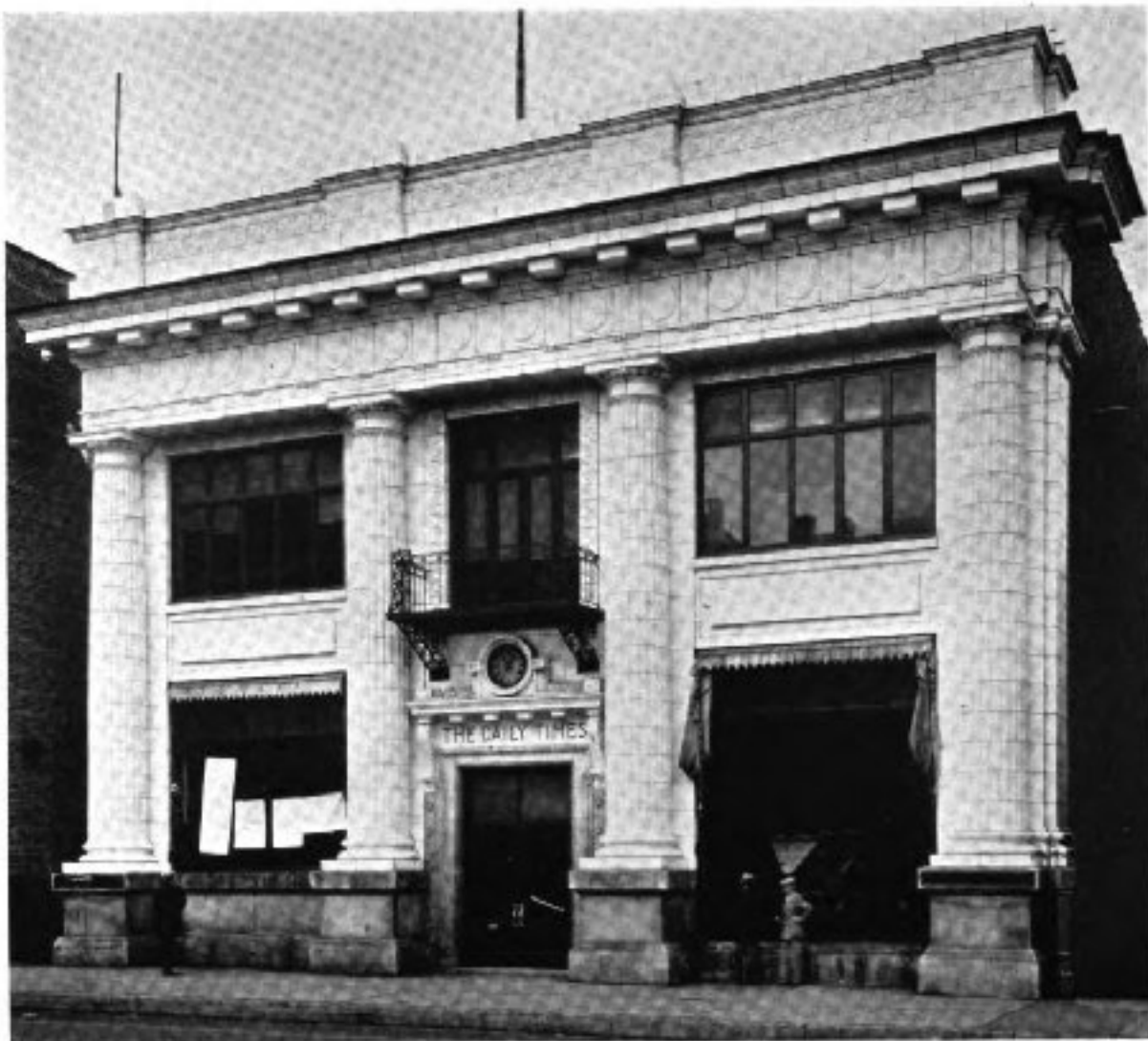
BUILDING OF THE DAVENPORT TIMES
