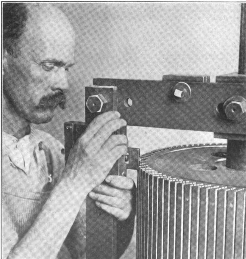
FIG. 8. MILLING NARROW WARD SLOTS
