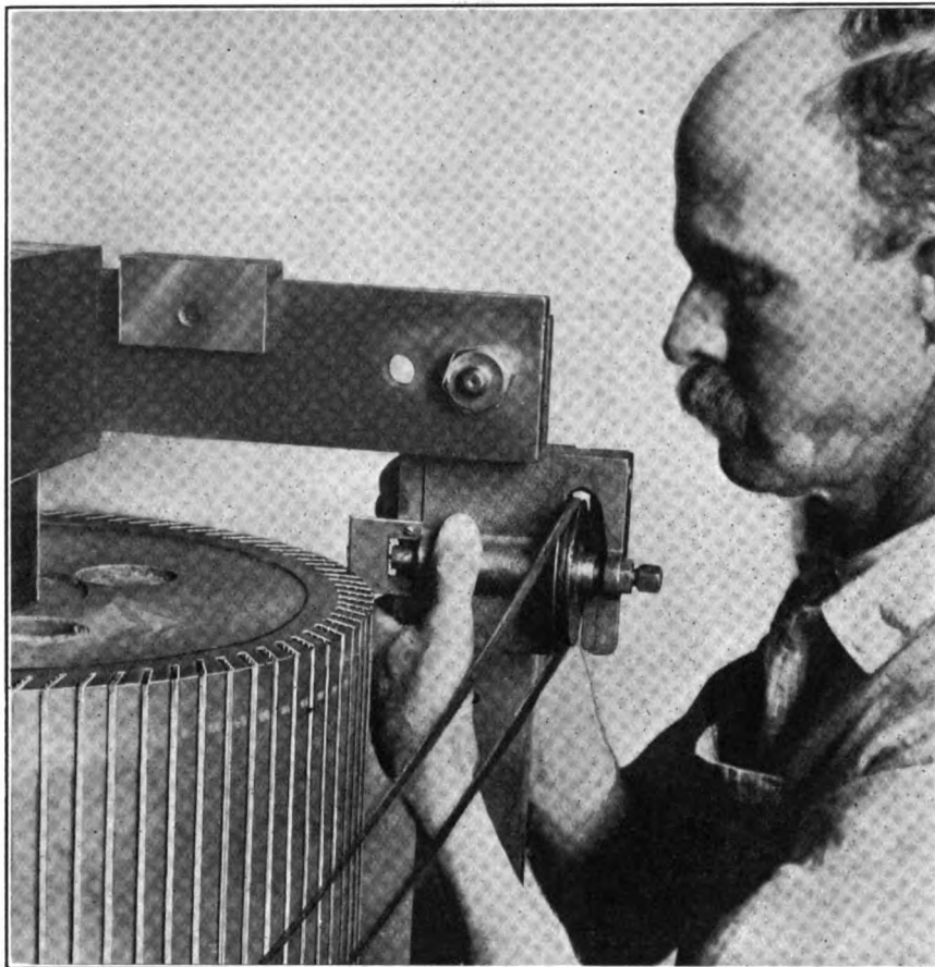
FIG. 7. MILLING NARROW WARD SLOTS
