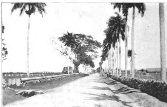
GENERAL VIEW OF WESTERN TROCHA.
