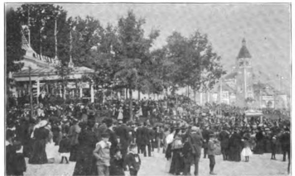
PENNSYLVANIA BUILDING ON LIBERTY BELL DAY.
