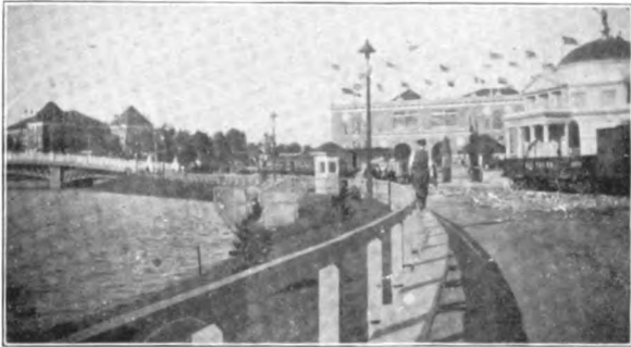
THE BRIDGE NEAR TRANSPORTATION BUILDING.
