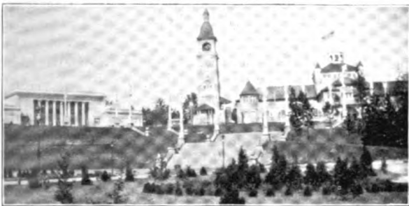
VIEW FROM THE PLAZA TOWARD CLOCK TOWER.
