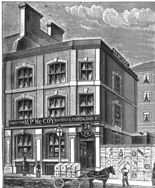
First building beyond Clerkenwell Road and the Underground Railway Opening.
