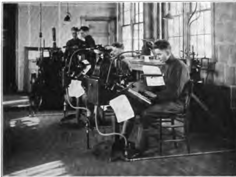
THE MONOTYPE SECTION, GENERAL HOSPITAL NO. 2 AT FORT MCHENRY, MARYLAND
