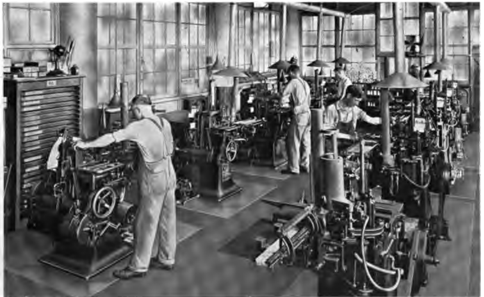
A CORNER IN THE MONOTYPE CASTING MACHINE DEPARTMENT
