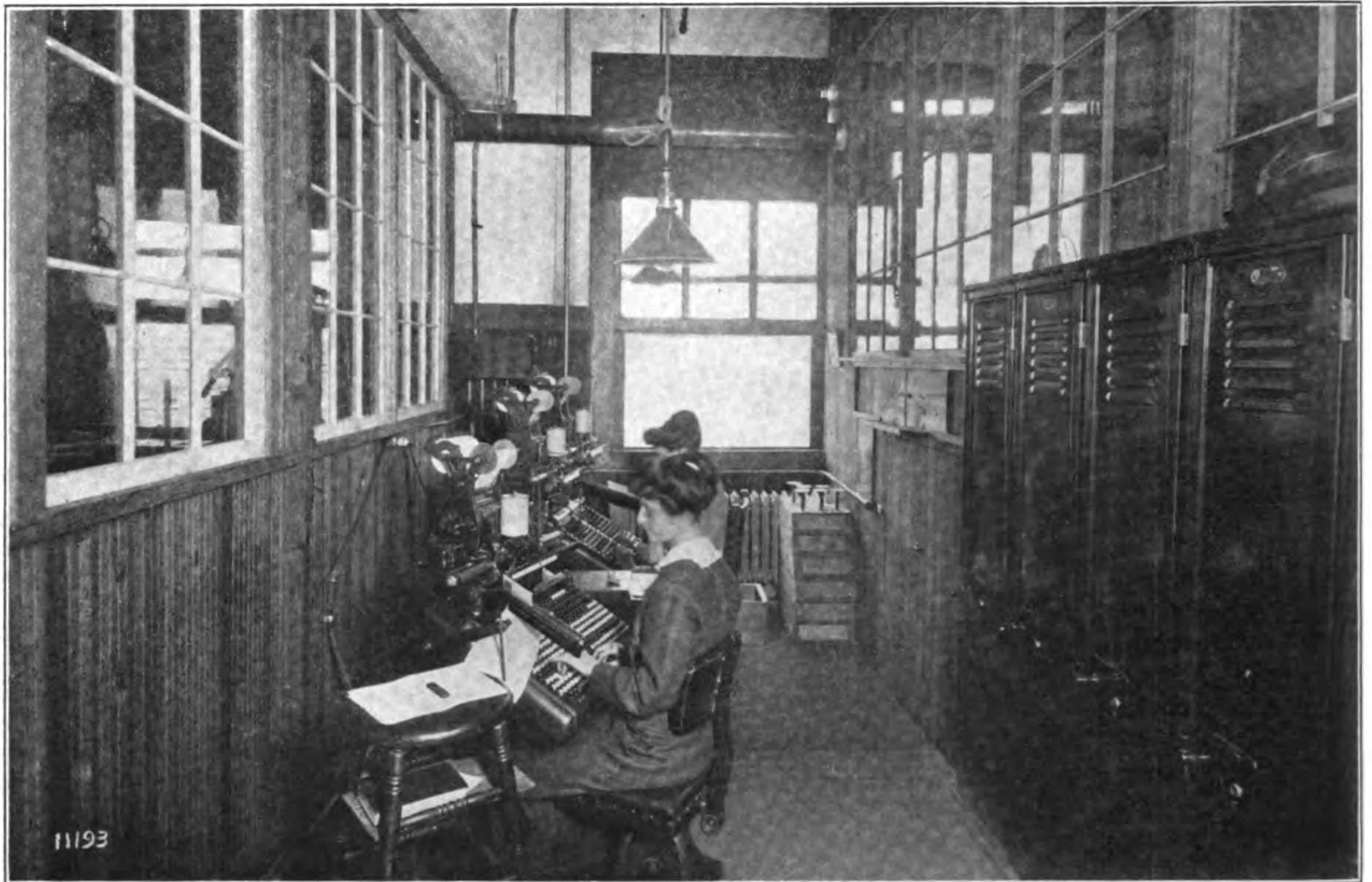
One of the secrets of getting a big output from keyboard operators is to give them ideal working conditions. Few plants afford better working quarters for operators than the Keystone Company. This room is well lighted, well ventilated, and is almost sound proof
