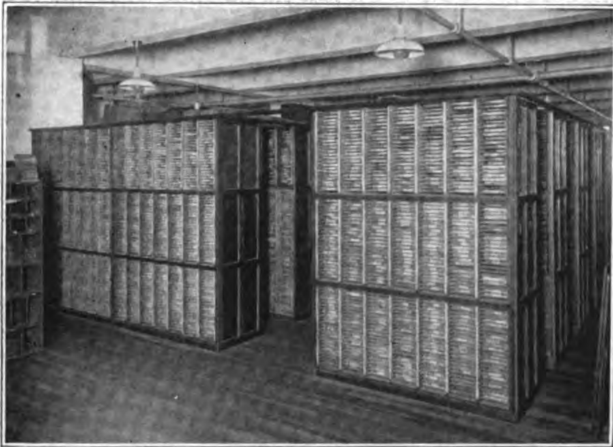
This view shows but a section of the Storage System built to take care of 50,000 tariff pages as well as numerous catalogs and directories
