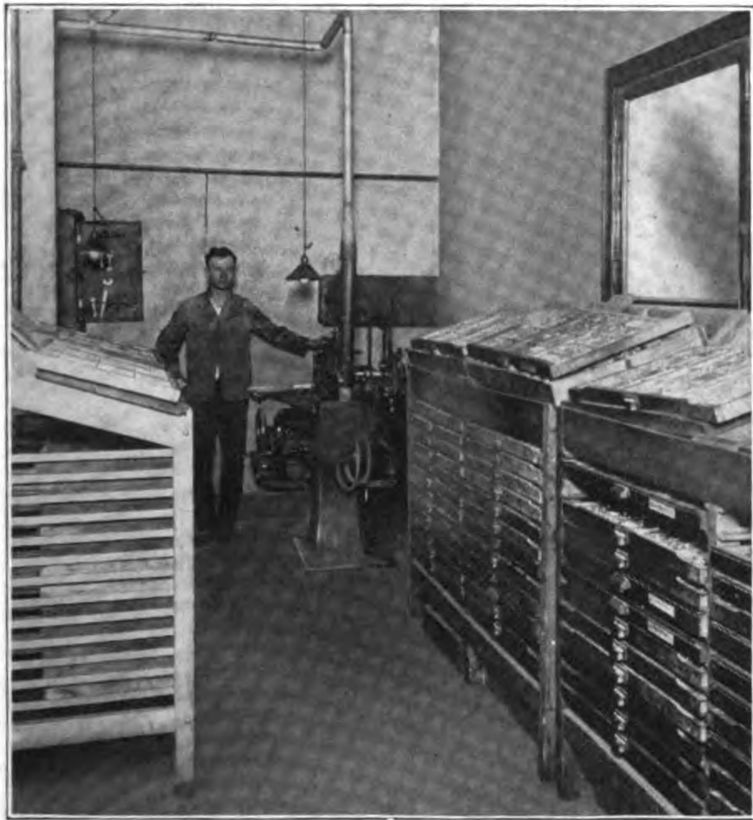
Caster Room at The Oklahoman , showing their Case Storage System. Full cases replace the cases in the Ad-Room that are running short of sorts
