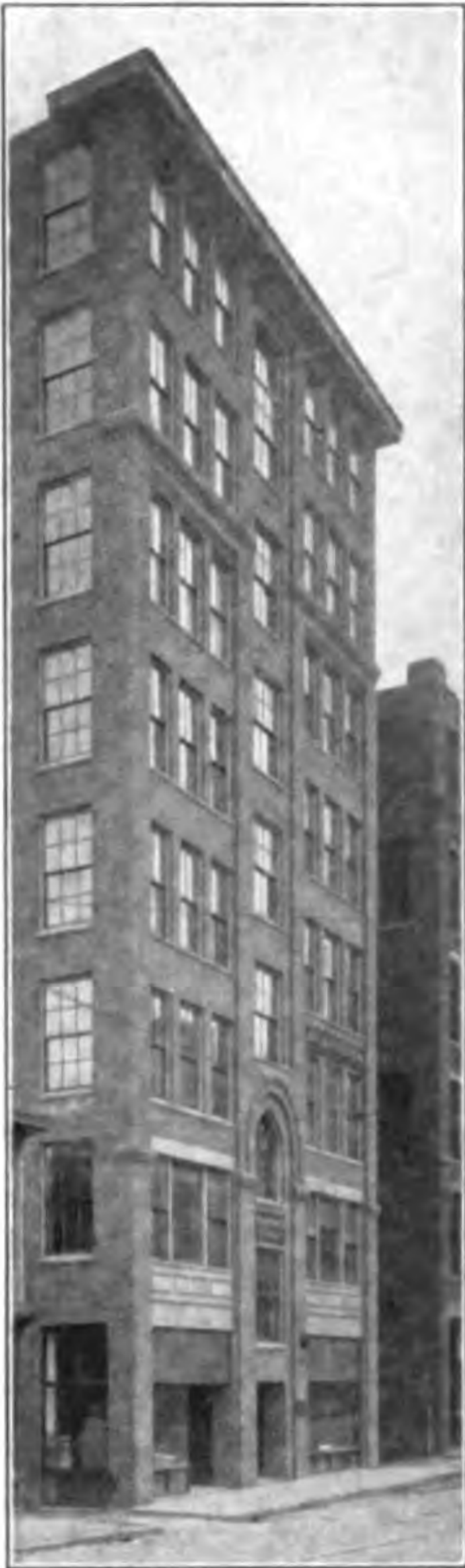
THE HERALD BUILDING HAVERHILL, MASS.
